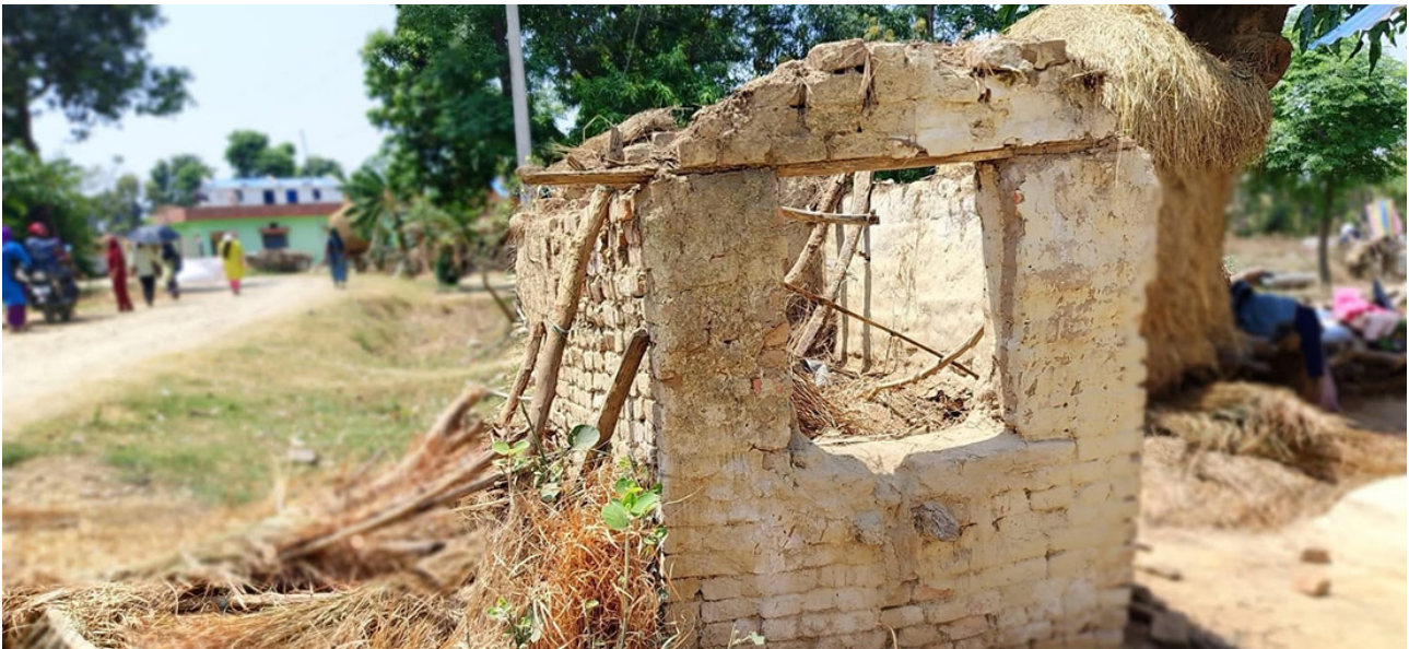
Chhaugoth Demolish at Dhangadi-12, Kailali
